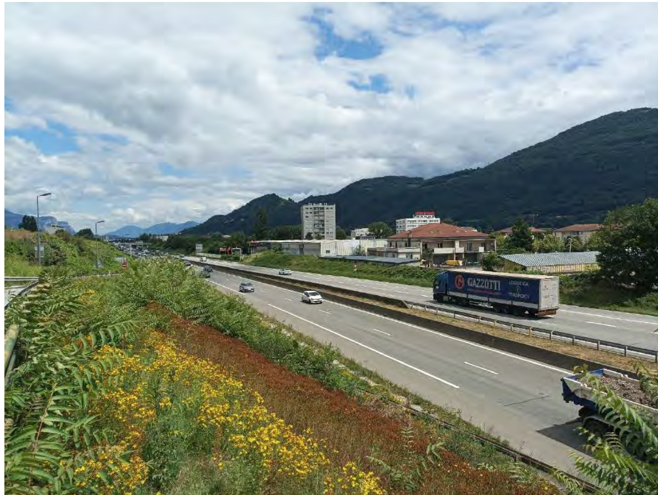
Figure 81 : Rocade Sud (N87)
